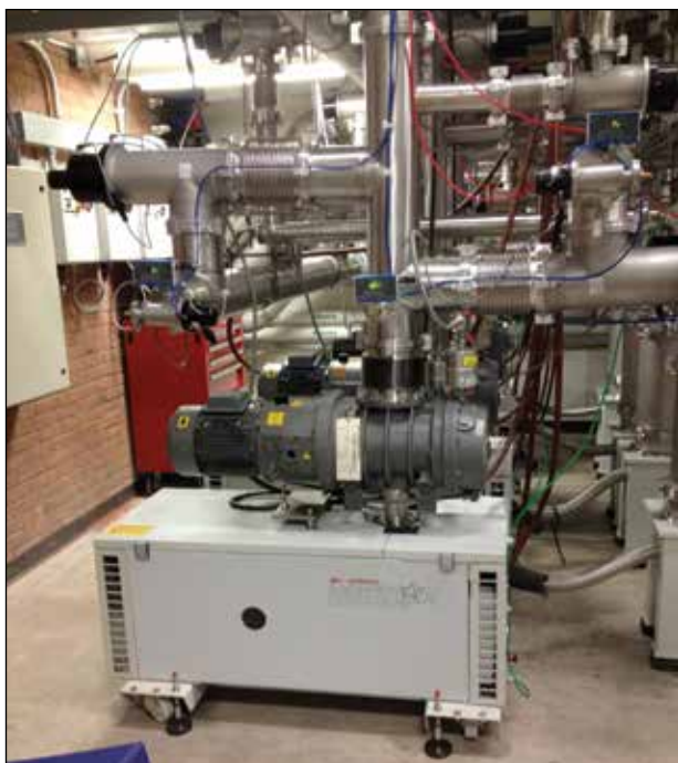
Figure 4.3 Typical mechanical pump with booster and pump-side vacuum manifold.
