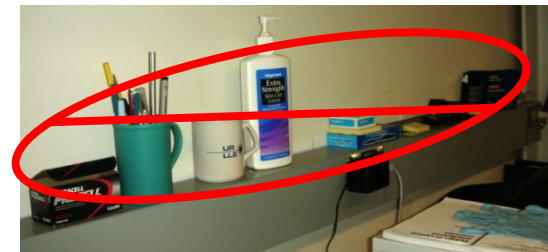
Raceway storage NOT OK
