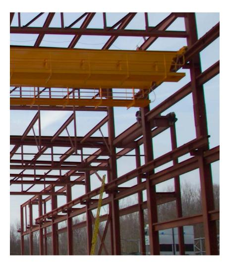
runway: an assembly of rails, beams, girders, brackets, and framework on which the crane travels
