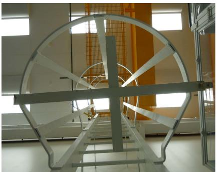
Unlock cage ladder access leaving the key in the lock as shown
